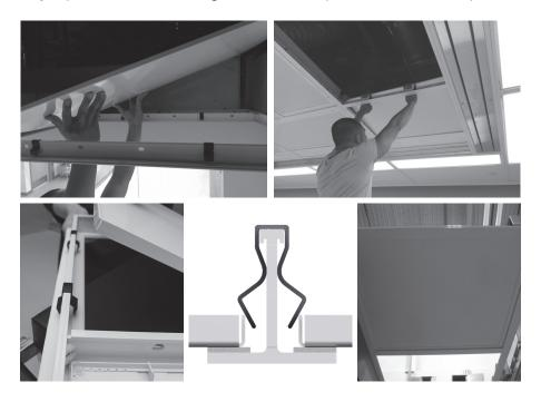
Figure 20: Ceiling Access Panel Installation
