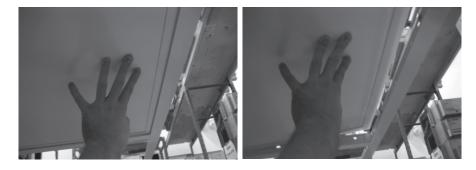
Figure 21: Access Panel Removal
